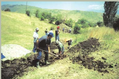
Excavation for a water supply pipeline at v. Dolgaec ▼
